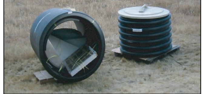
Lowering the tank into the ground.
