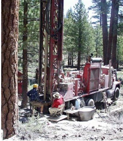
EarthScope is installing borehole strainmeters, seismometers, and GPS stations across the Pacific Northwest. Sensitive enough to record events a world away, they will tell us much about the Earth's interior and how different regions are changed by plate tectonics.
